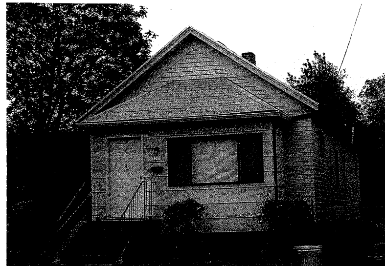
West Clinton home after renovation by REACH.
