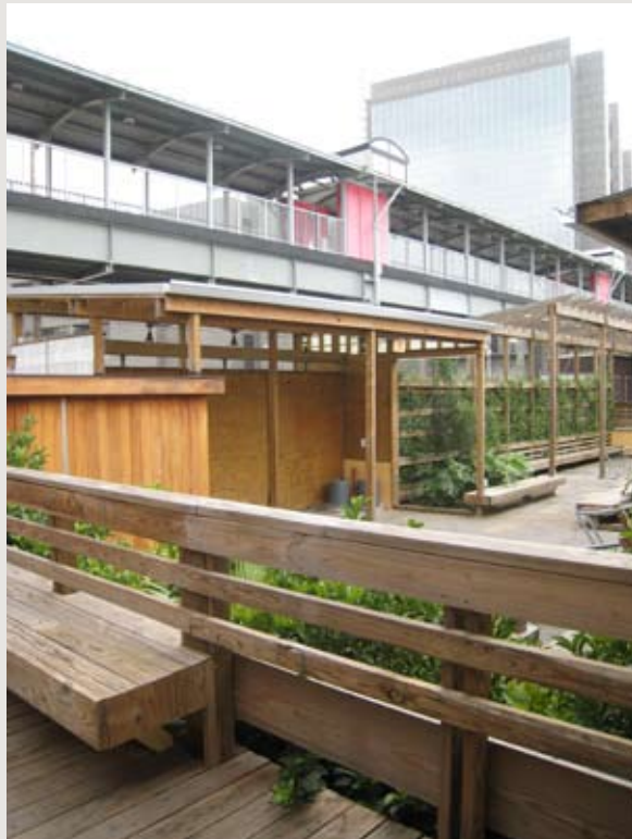
Entrance to Rebuild Center with pedestrian sky bridge and medical center in background
